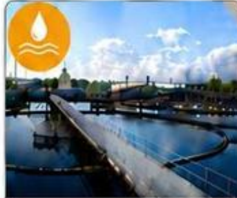
WATER TREATMENT PLANTS
